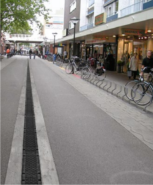
Loading and unloading zones
