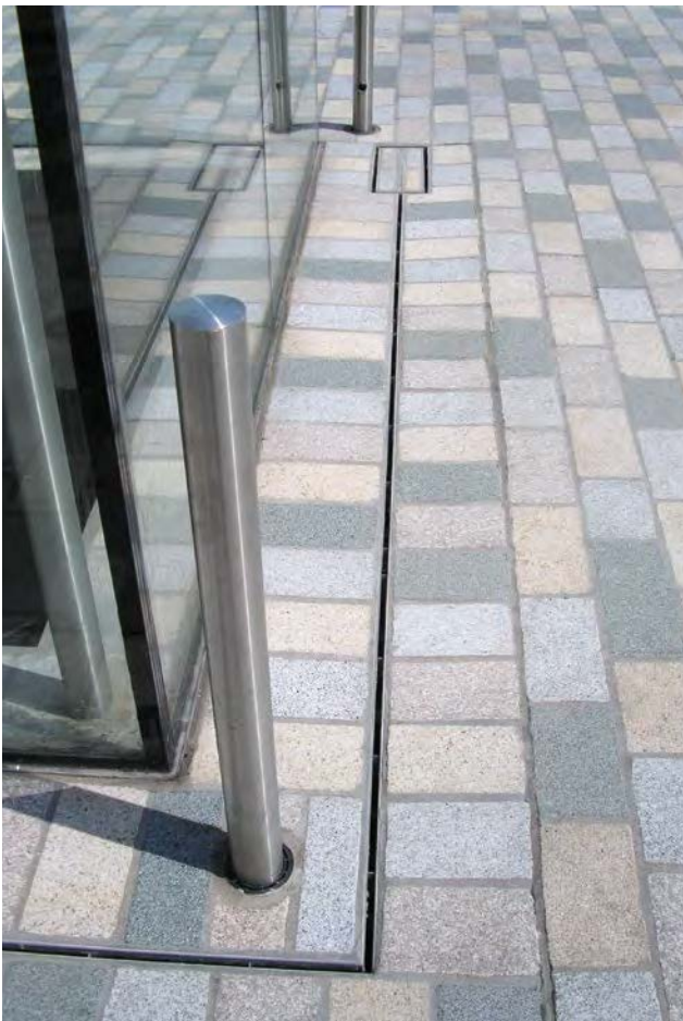
Town hall square in Esch-sur-Alzette, France
